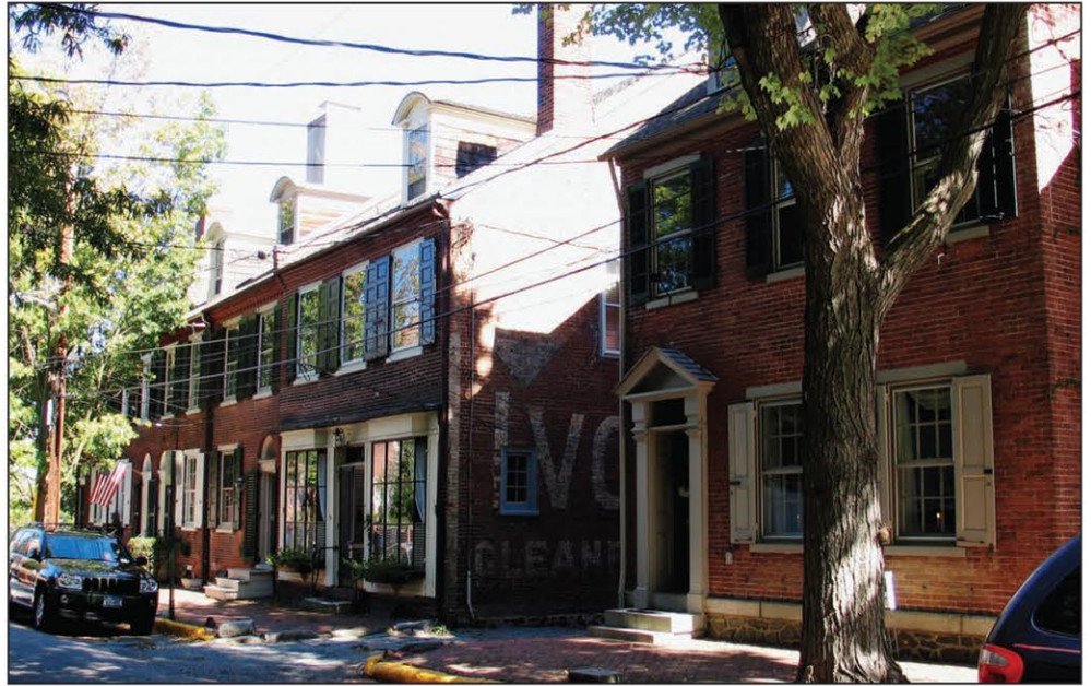
Side view of the Stage Tavern, also known as Bouldens Store building, in middle of photograph.
