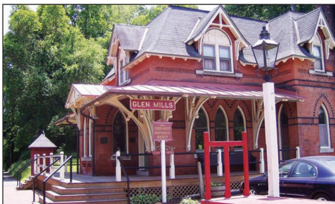
The Glen Mills train station.
